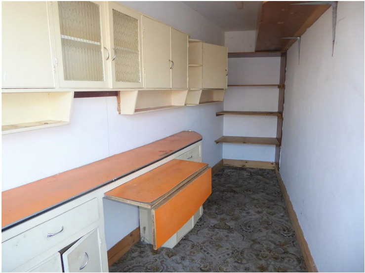
Wall and floor mounted unit, power and lighting.
